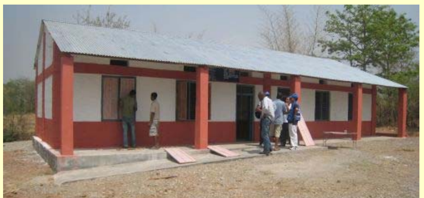
Two more classrooms of Balapur Secondary School constructed with the support of QIPSI
